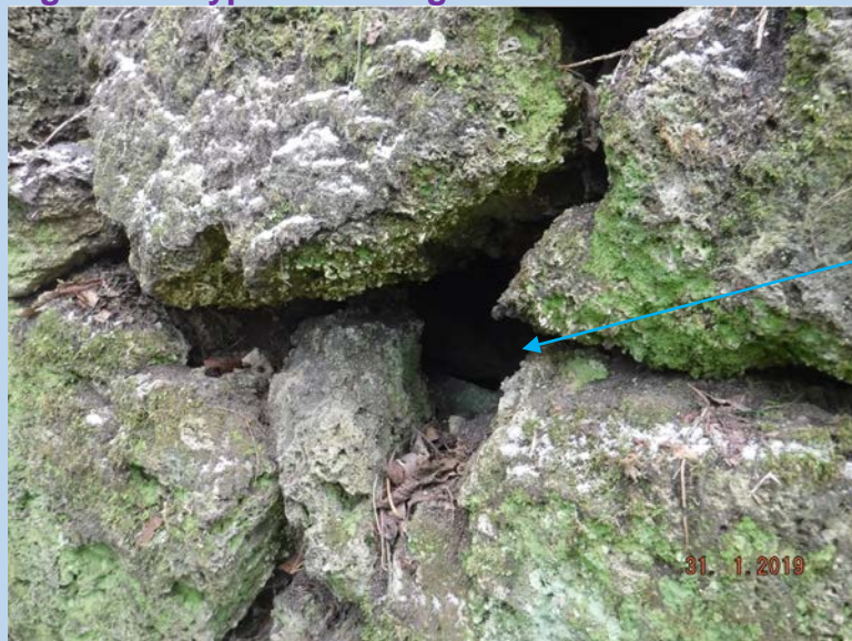
Figure 3 – Typical Voiding of Wall and Foundations
