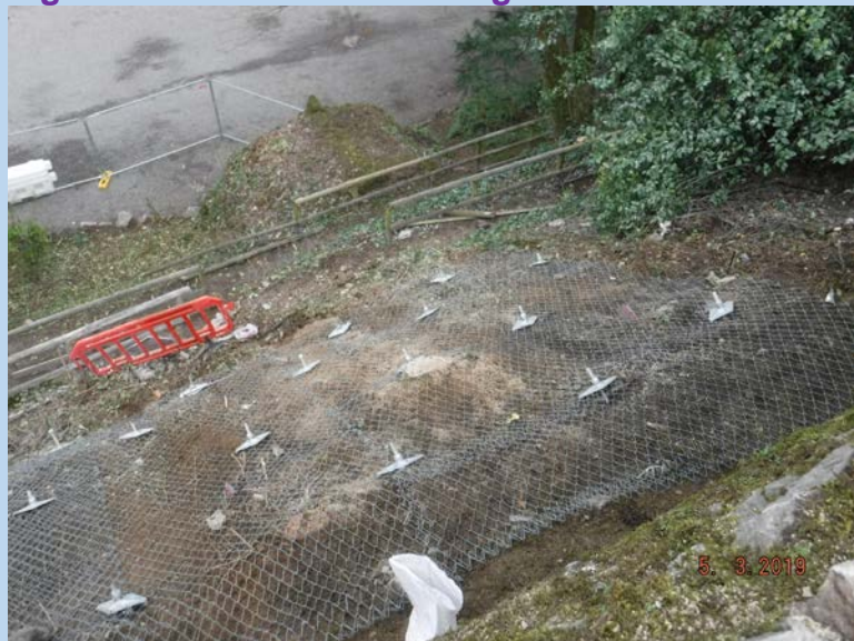
Figure 4 – Soil Nails to Strengthen Embankment
