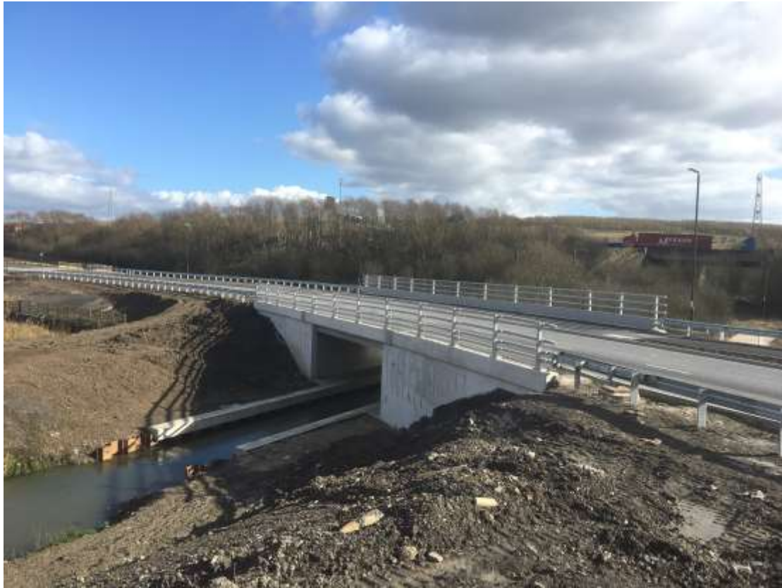
The new Seymour Link Road bridge over the Doe Lea river
