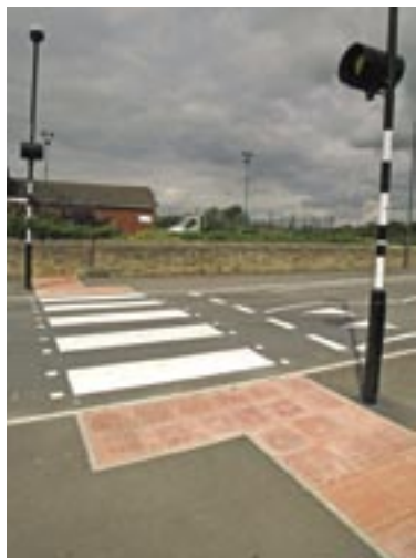
Pedestrian crossing improvement at Belper.
