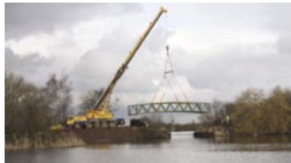
Trent Valley Greenway cycle bridge installation over the Erewash outfall.
