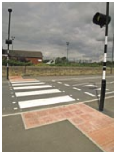
Pedestrian crossing improvement at Belper.
