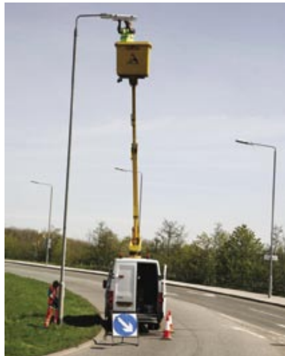
Street lighting maintenance.
