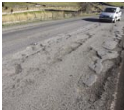
Brierlow Bar carriageway repairs. Before.
