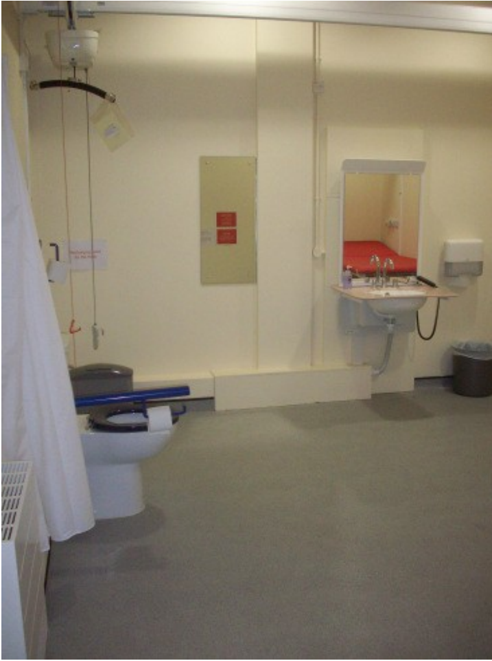
Hoist, toilet and rise and fall unit
