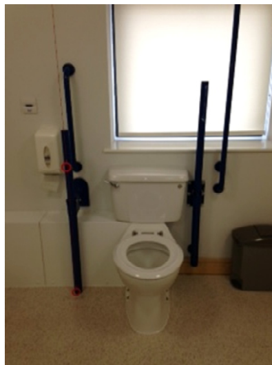
The toilet with space either side for assistance
