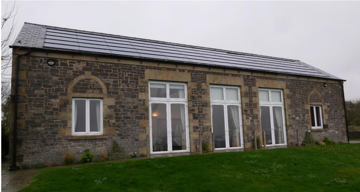
Over Haddon Village Hall, Derbyshire: Solar PV and air source heat pumps, within the Peak District National Park and on the edge of the Over Haddon Conservation Area. Image with permission of Over Haddon Village Hall.
