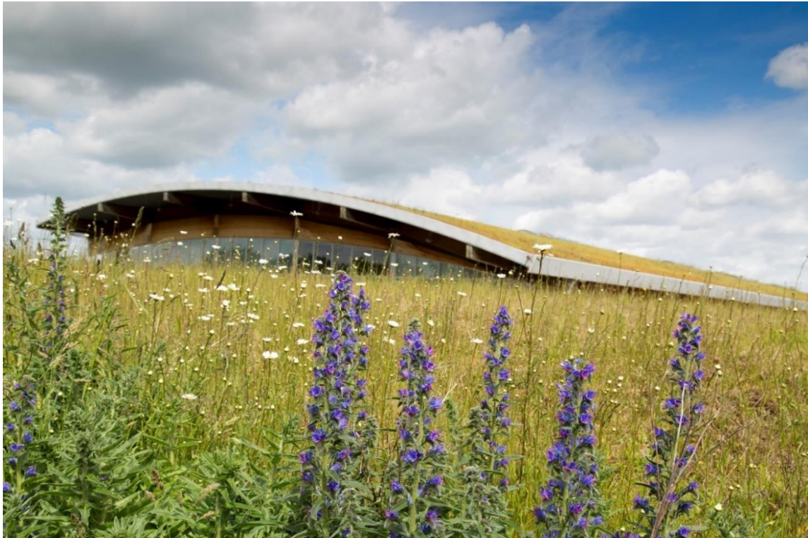
Adnams Distribution Centre, Reydon. Wildflower meadow planting, green roof, Sustainable Drainage systems and low embedded energy building materials. Image provided by Adnams Plc.
