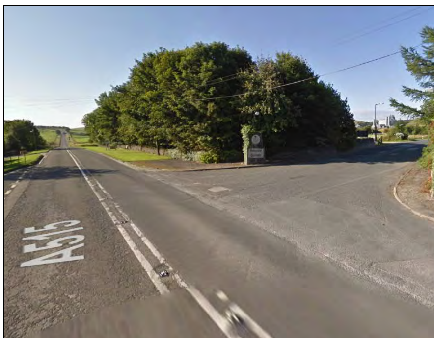
Figure 5.10: Hindlow Quarry site access (© Google)
