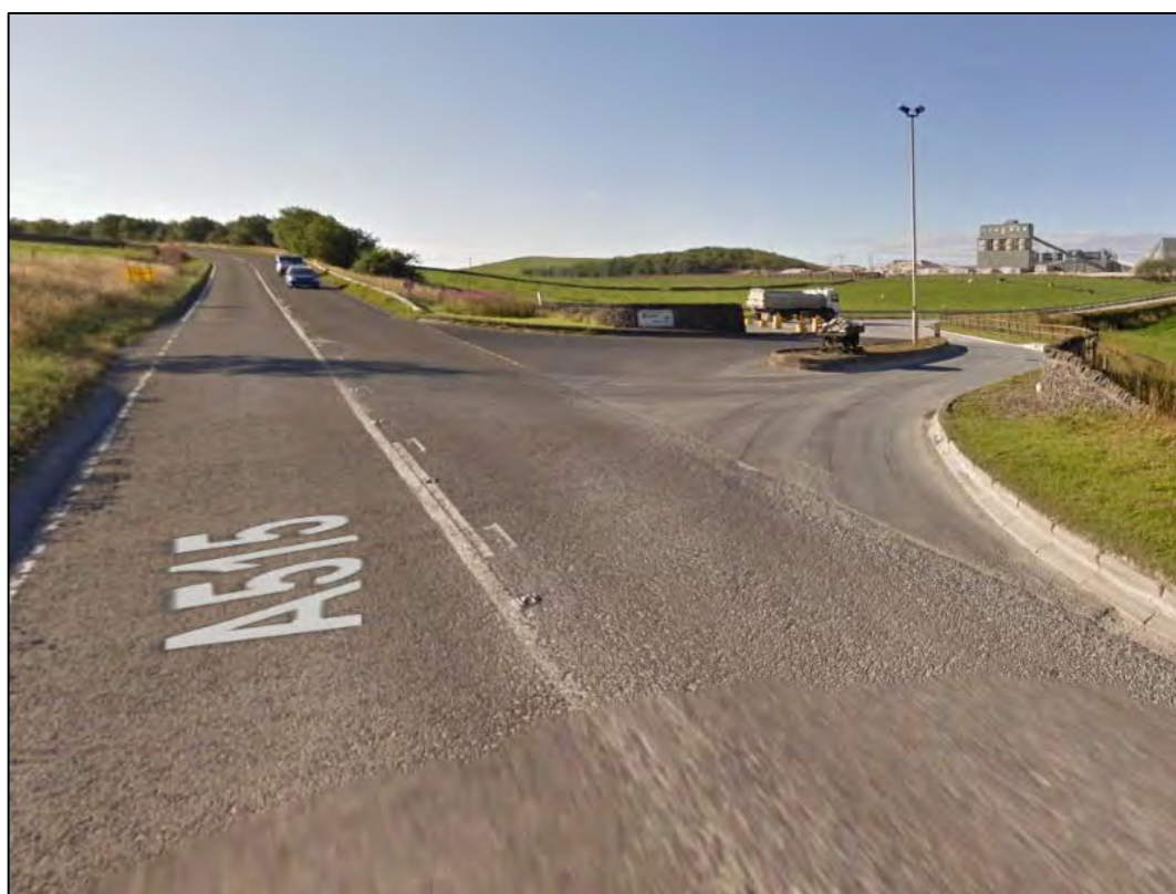
Figure 5.11: Dowlow Quarry site access (© Google)
