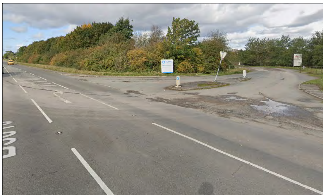
Figure 5.36: Elvaston Quarry site access (© Google)
