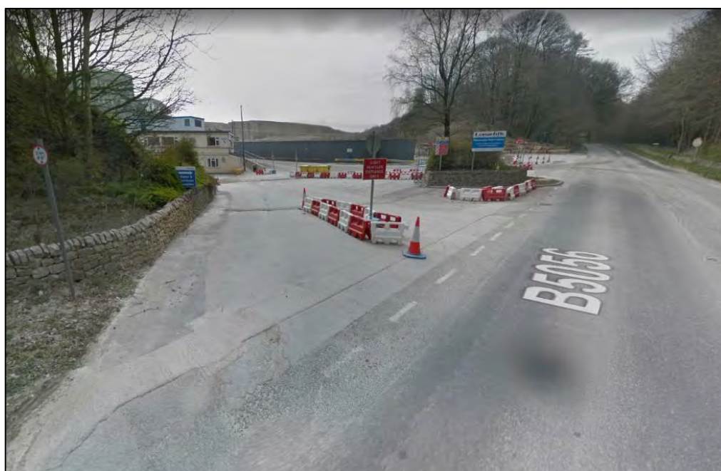
Figure 5.15: Brassington Moor site access – Light Vehicles (© Google)
