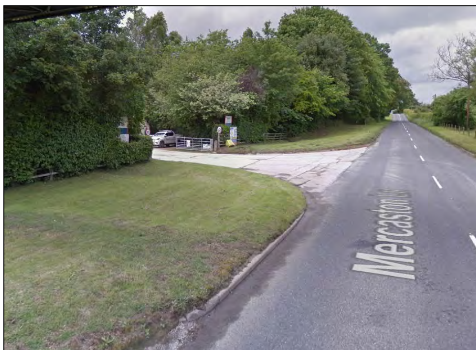
Figure 5.25: Mercaston Quarry site access (© Google)
