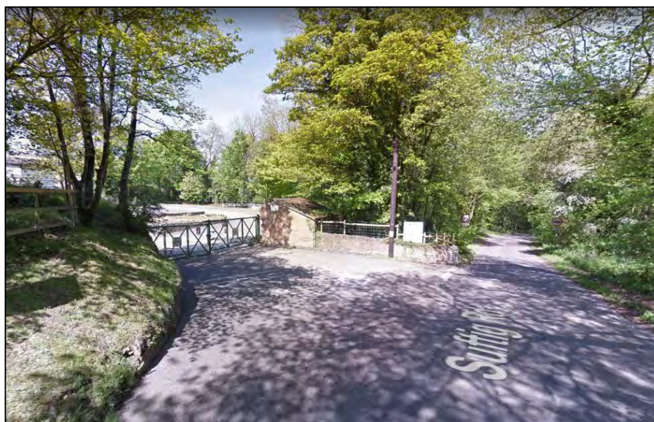
Figure 5.28: Bolsover Moor site access (© Google)
