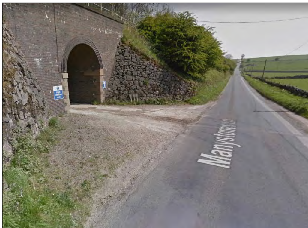
Figure 5.13: Bone Mill Quarry secondary access – light vehicles only (© Google)
