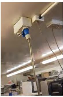
The electricity and gas supply are high up and can be easily turned off and back on.
