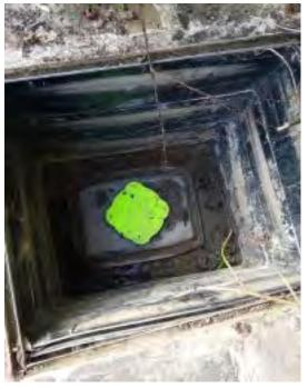
The culvert running underneath the house now has two non-return valves.
