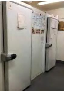
Cold stores have fitted rubber seals but in addition marine ply is sealed to the fronts.
