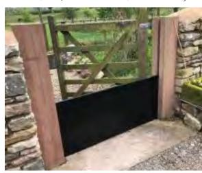
Marine ply slot-in barriers put behind the gates in the wall.
