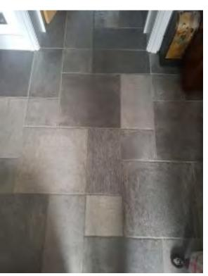
Tiling in the ground floor above insulation and underfloor heating.
