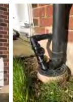
${\it Electric sockets further up\ the\ walls,\ barriers\ to\ all\ external\ doors\ and\ non-return\ valves\ fitted.}$
