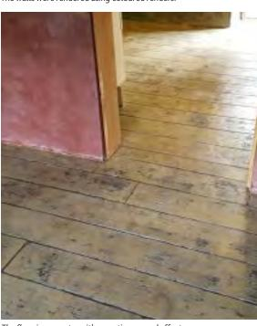
The floor is concrete, with an antique wood effect pattern, and sealed to give a gloss finish.
