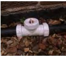
Non-return valve in pipework, to prevent backflow.
