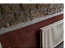
The walls were rendered on top of the membrane, using coloured renders
