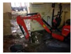
The rebuild involved excavating and 'tanking' the whole of the ground floor
