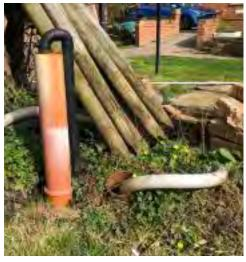
Rainwater runs through a series of French drains into a large sump into which a strong pump is fitted which pumps the water outside the garden boundaries.
