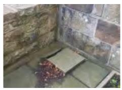
Sump created, into which powerful submersible pump can be dropped when flooding commences.
