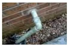
Brickwork sealed using special cement.
