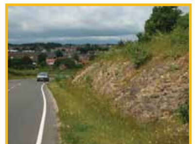
Retention of exposed geology adjacent to new road with species rich grass verge
