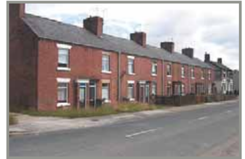
Red brick mining terrace
