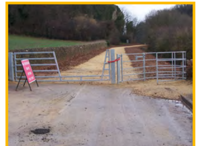
Crushed magnesian limestone surfacing and simplified access arrangement
