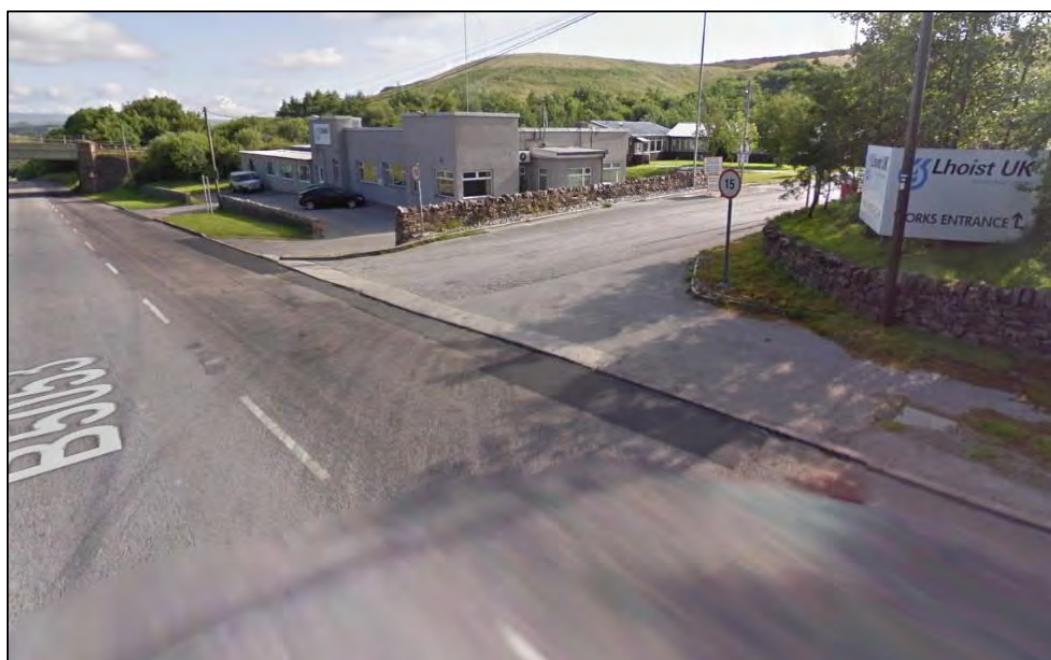
Figure 5.9: Brierlow Quarry site access (© Google)
