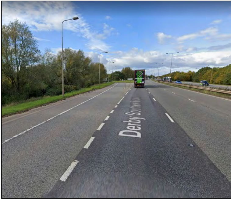
Figure 5.37: Shardlow Quarry site access – A50 off-slip (© Google)
