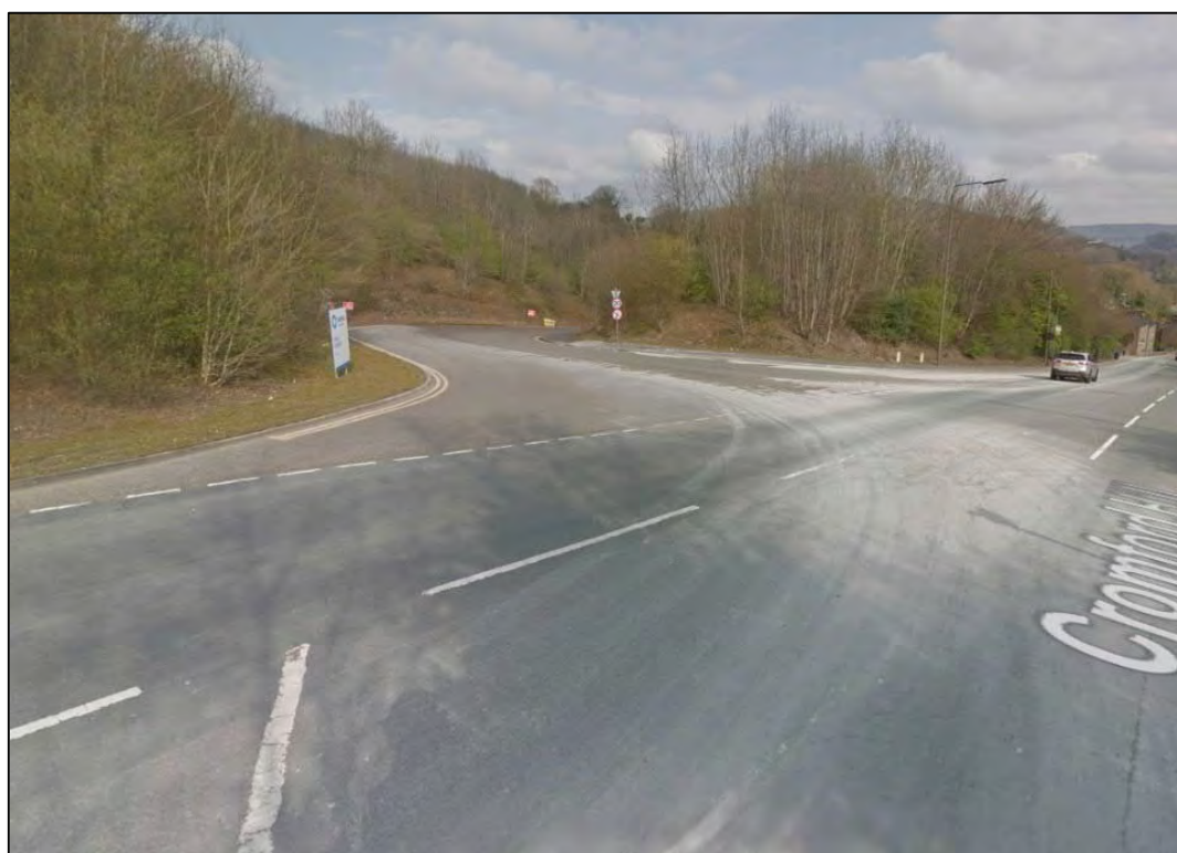
Figure 5.23: Slinter Top Quarry site access (© Google)
