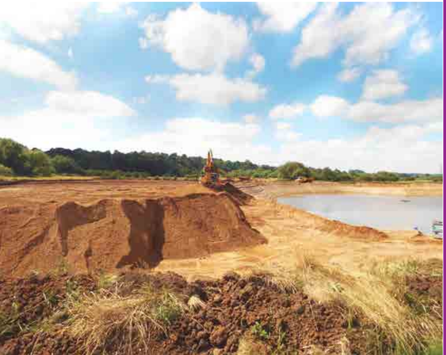
Shardlow Quarry - sand and gravel extraction
