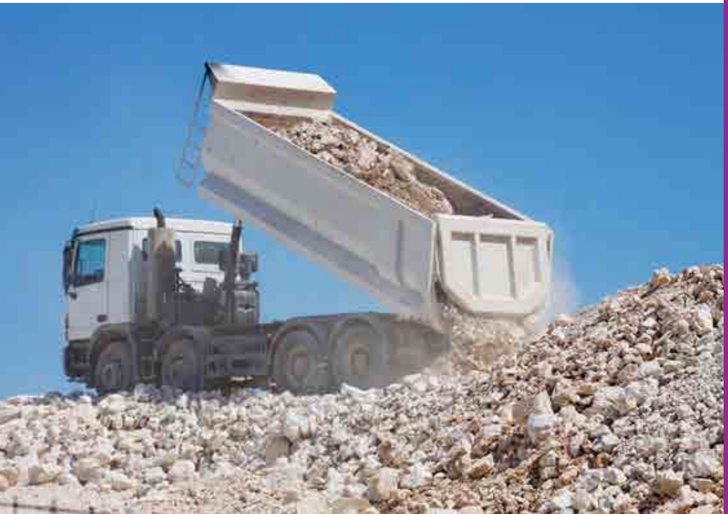
Tipper truck unloading crushed rock
