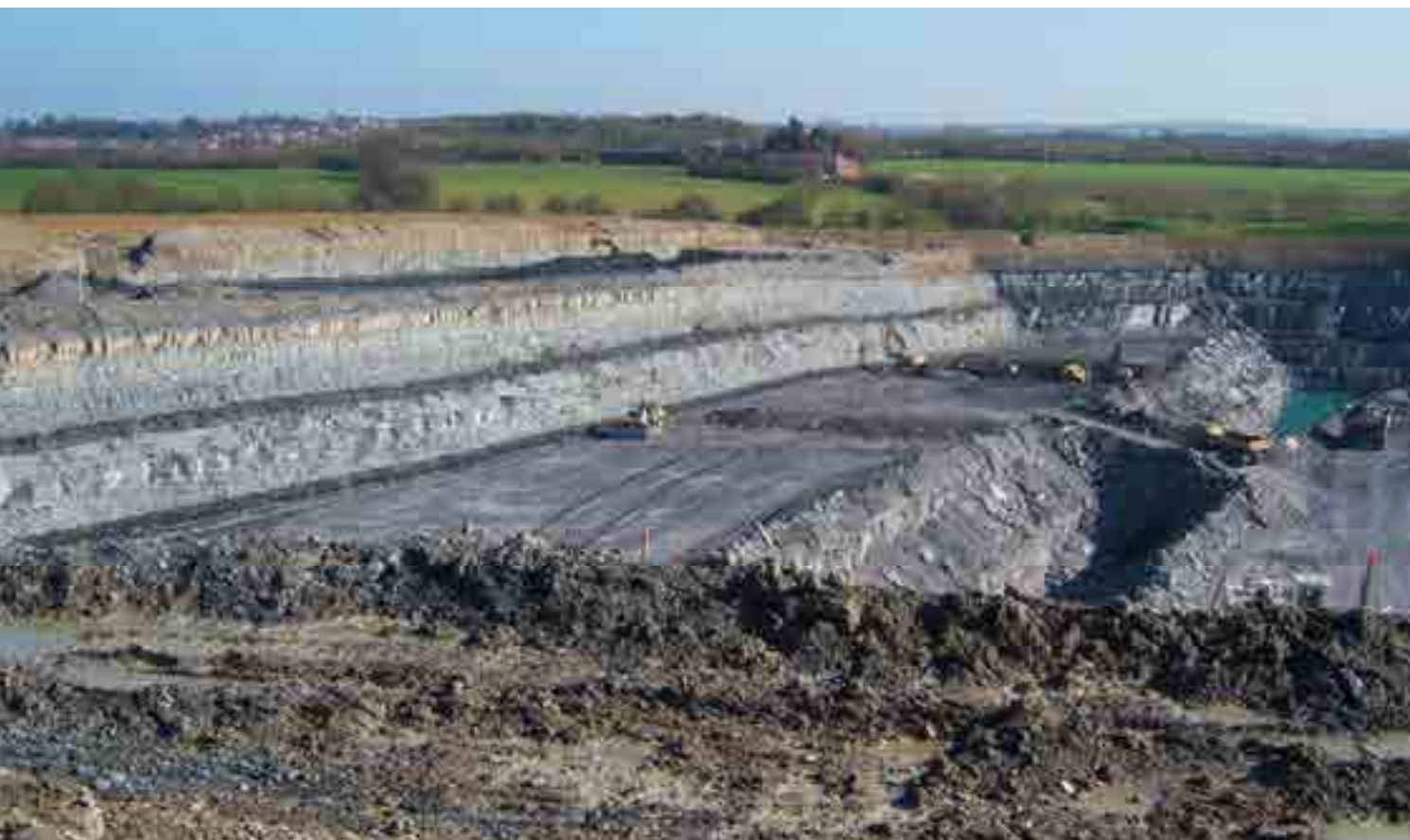
Lodge House - pre soil replacement 2011
