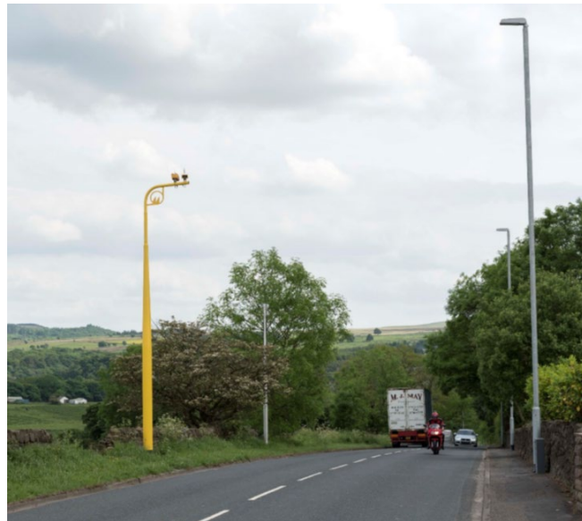
Photograph showing standard high visibility passively safe column in Traffic Yellow colour. This is the most common configuration with more than 400 columns like this across the UK.
