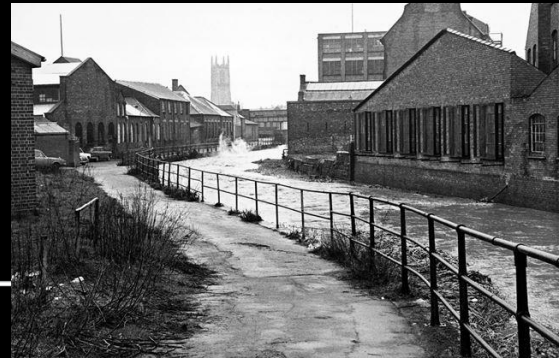
1977, Markeaton Brook Walkway, facing towards Ford Street
